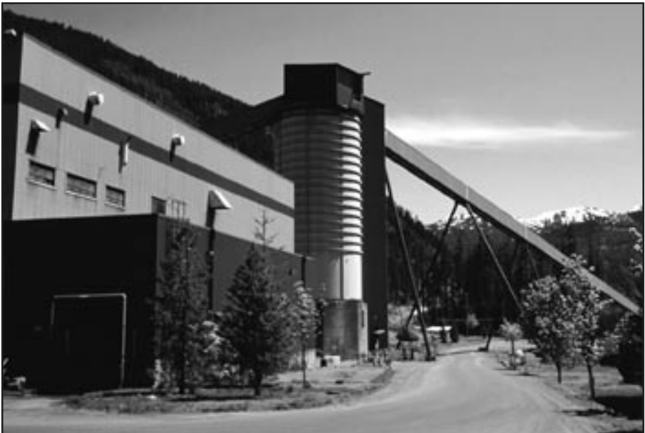
The ore conveyor and mill at Boliden-Westmin Myra Falls mine.
